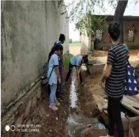
Drainage cleaning in Hasampura village
