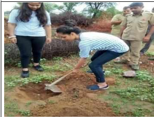
Students constructing the compost pit
