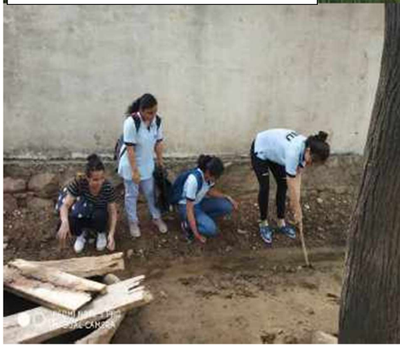
Drainage cleaning in Hasampura village
