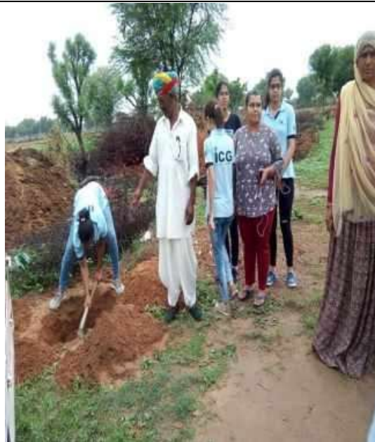
Villagers giving direction for constructing compost pit
