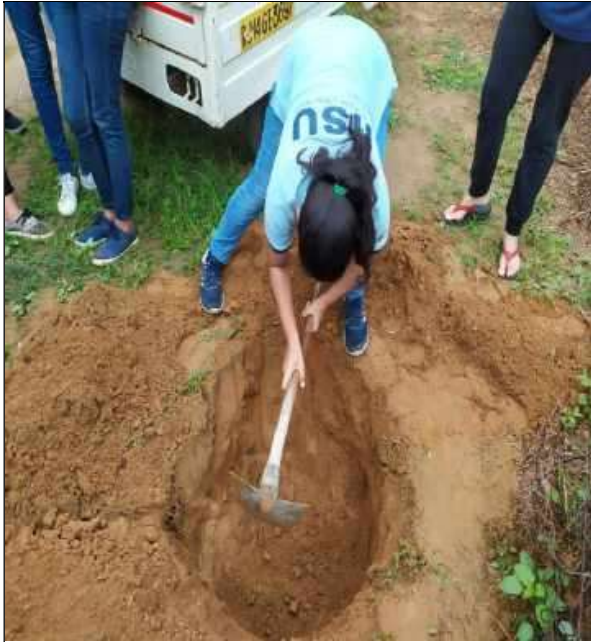
Students constructing the compost pit
